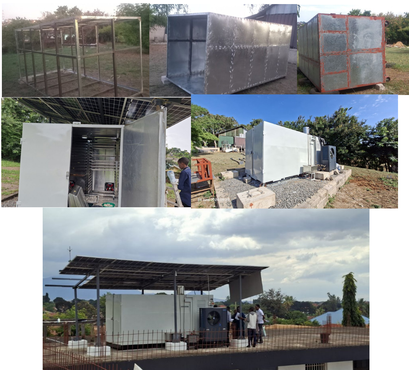
Journey of SS2 dryer from its design, fabrication, testing to its actual installation site
